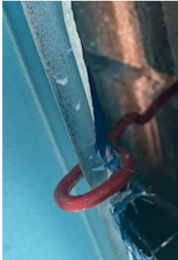
**Figure 1: Tie fixing on lip of steel stud**
